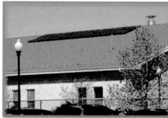
Reed Intermediate School Solar Panel Project
